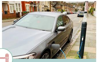
The Royal Borough of Greenwich has upgraded some lampposts to LED lighting, and equipped some with a Central Management System (CMS) to gather a wide range of data. Some of the lampposts also have EV charging points in their poles and provide connectivity for smart parking sensors.
